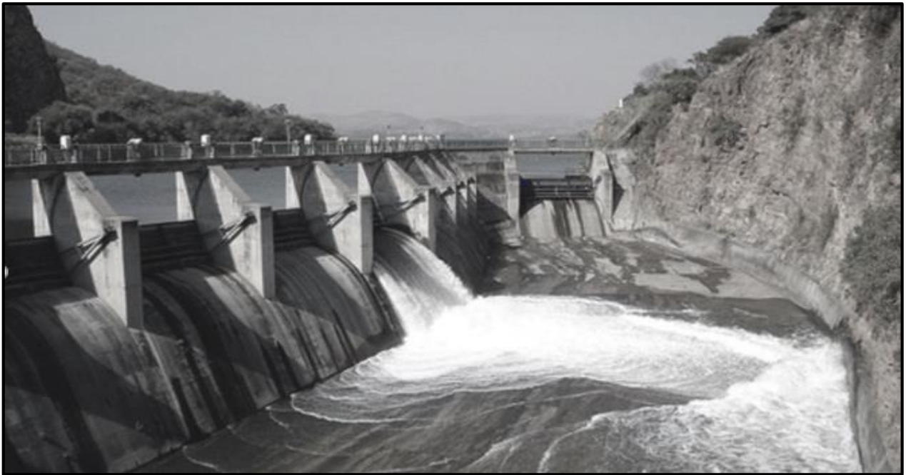
FIGURE 3.6: HARTBEESPOORT DAM WALL
